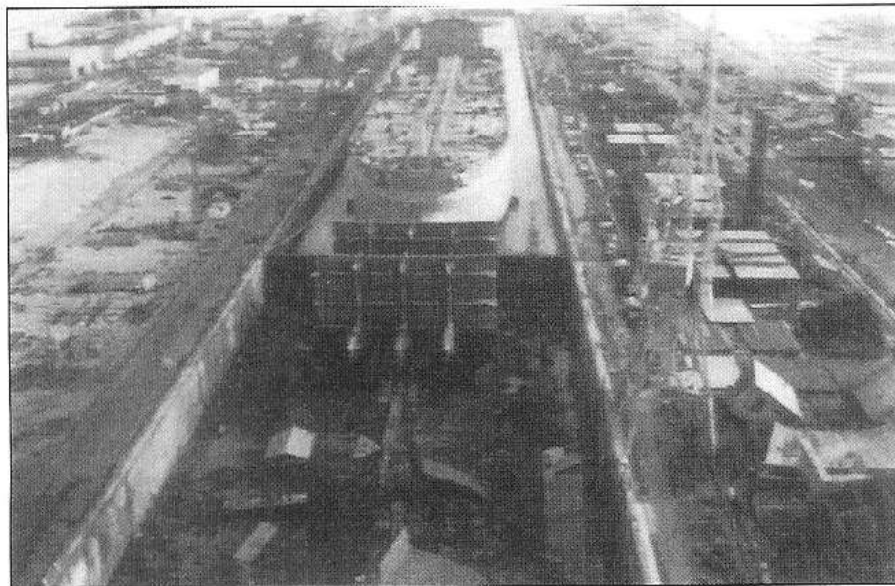
Fig. 5: The docks, again in operation, after the rehabilitation
